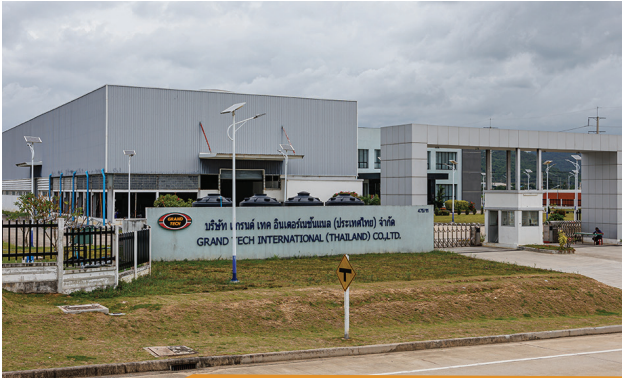
Grand Tech International (Thailand) Co.,Ltd. Si Racha District, Chonburi
