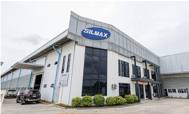
Silmax Sealing Solution Co.,Ltd. Pluak Daeng District, Rayong
